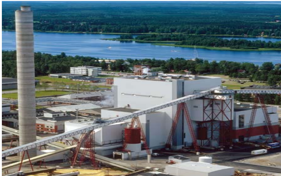
Figure 3.4 Alholmens Kraft biomass power plant, Pietarsaari (Finland)
