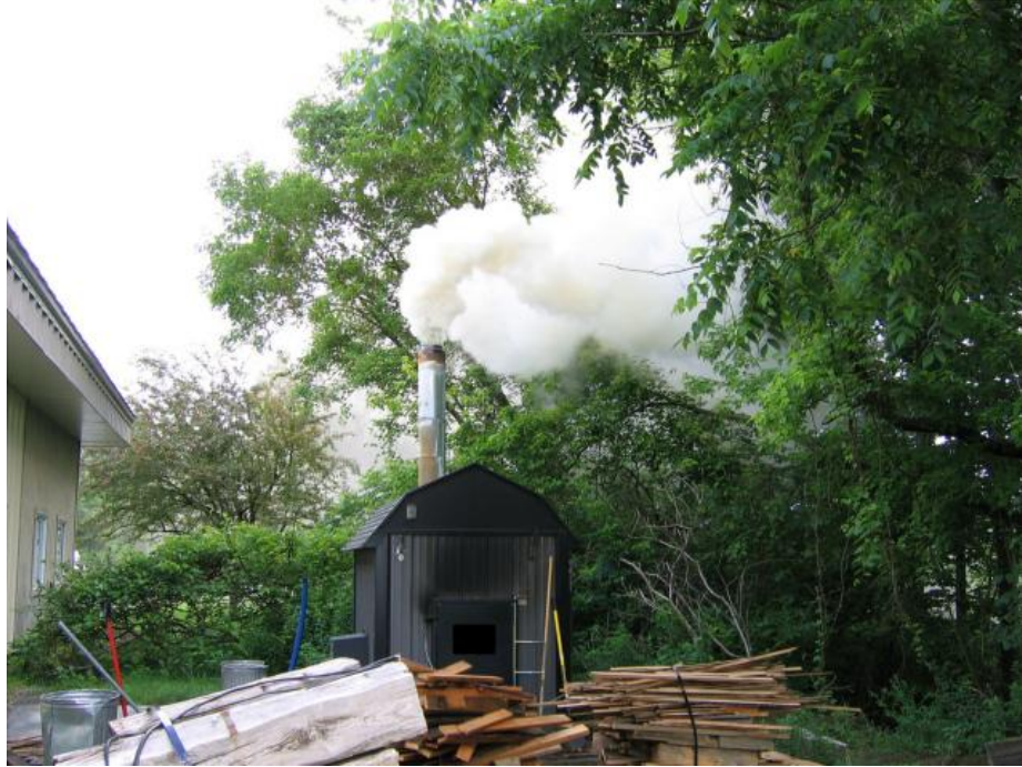
Figure 2. Outdoor wood boiler. Photo credit Phil Etter; photo borrowed from Burkhard, 2013. 16
