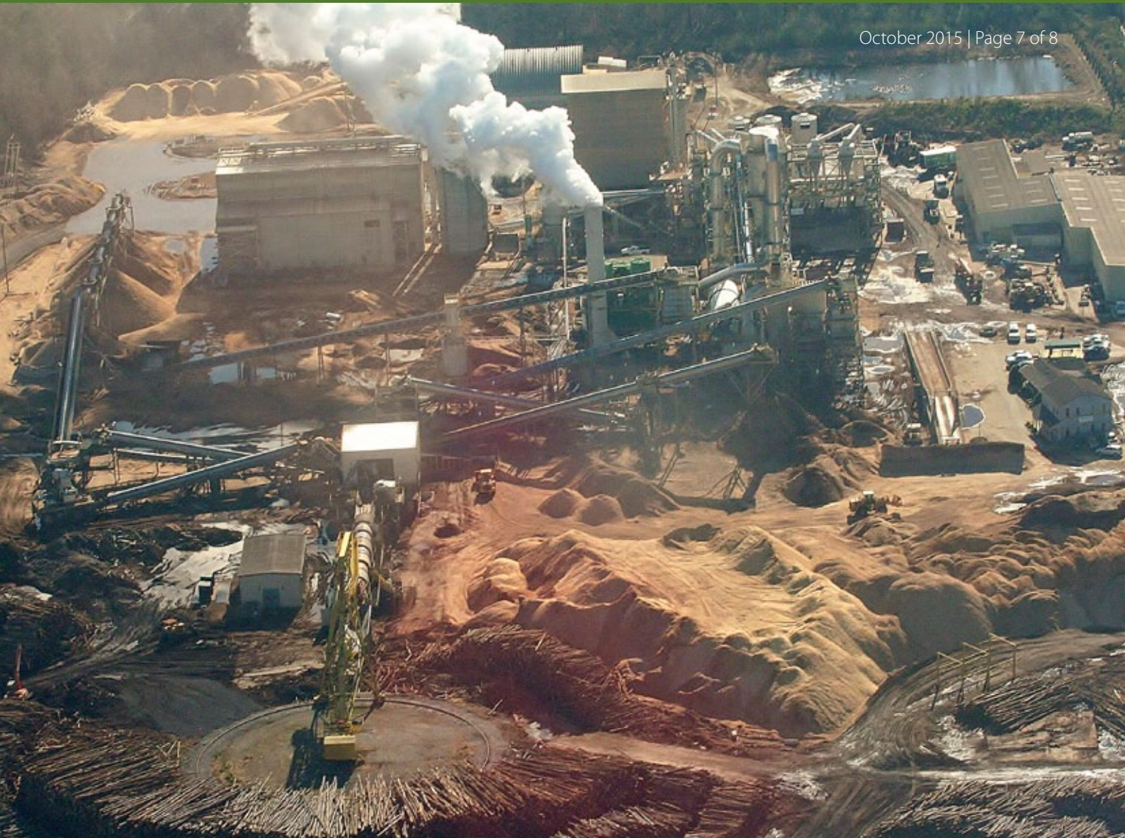
Enviva's facility in Ahoskie, North Carolina. Wood cut in US forests is converted into pellets here before being transported to the Drax power plant in the UK. Photo: Dogwood Alliance
