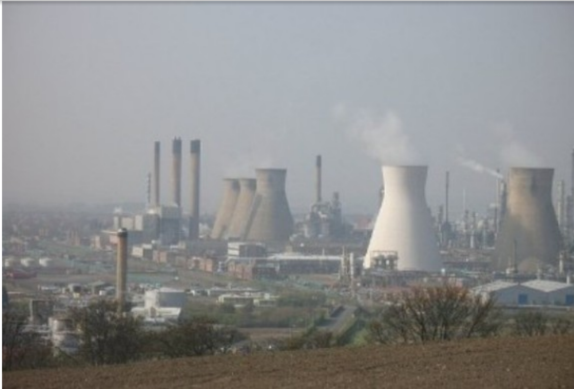
Grangemouth and its oil refinery, Photo: Richard Webb, www.geograph.org.uk/photo/1233455
