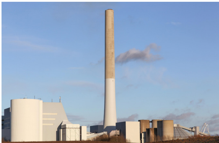
Ørsted Studstrup Power Station in Studstrup, Denmark.
