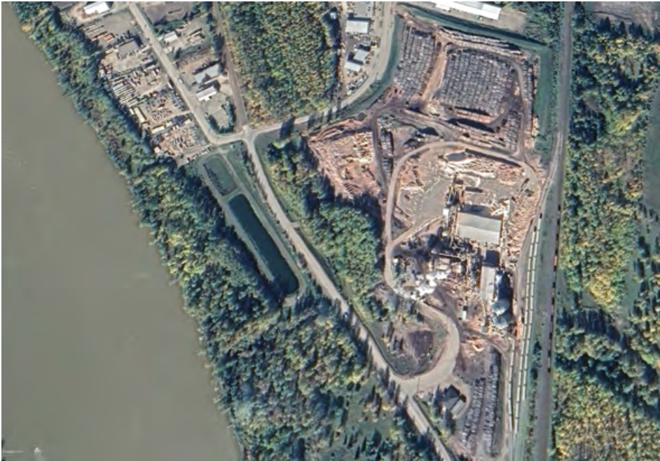
Figure 4: Pacific Bioenergy Pellet Mill, Prince George, BC. Image sourced: 2020 Google, CNES / Airbus.
