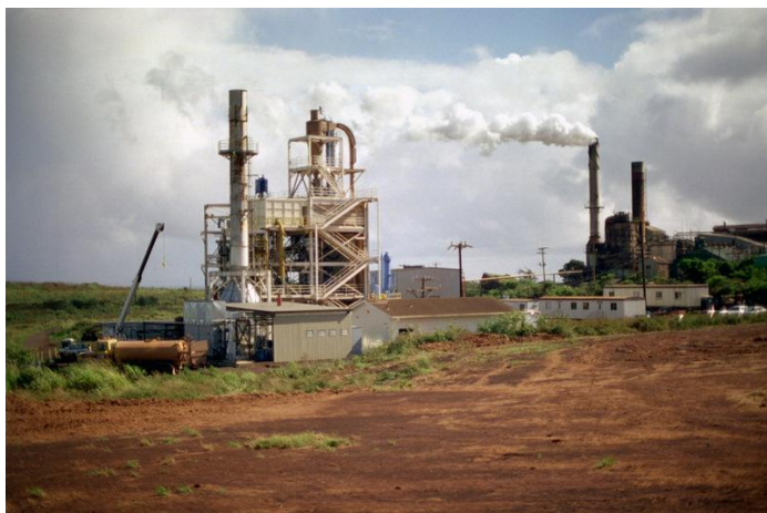
Figure 1. Biomass gasifier in Paia, Maui, Hawaii. This facility operated for a time in the 1990's and used sugarcane bagasse as fuel. Photo credit: Richard Bain, National Renewable Energy Laboratory.
