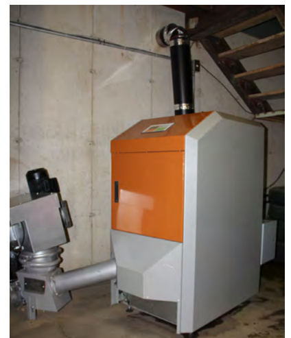
Figure 11. First Made-in-NY residential wood pellet boiler by EvoWorld. (Courtesy of EvoWorld)
