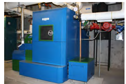
Figure 10. First Made-in-NY commercial high-efficiency wood pellet boiler by Advanced Climate Technologies. (NYSERDA photo)
