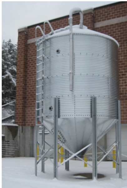
Figure 6. Bulk pellet storage silo. (Courtesy of ACT Bioenergy)
